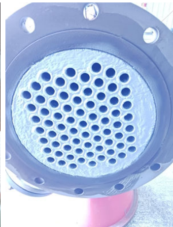
Application of Belzona 1391T Grey completed
