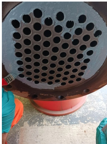
Application of Belzona 1391T Blue
