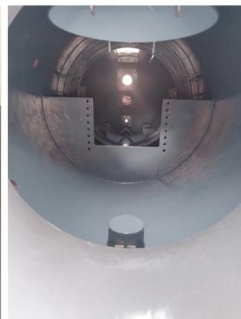
A second coat of Belzona 1391T was applied to ensure durable, long-term protection.
