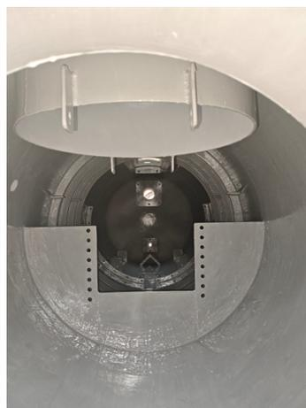
The damaged areas were then treated with a first coat of Belzona 1391T.
