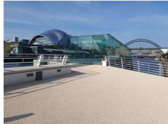
1mm of Belzona was applied and blended with aggregate
