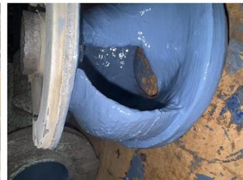
2nd Coat of Belzona 1321 Applied
