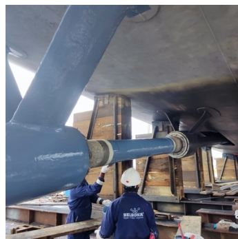
Application of the first coat of Belzona 5821
