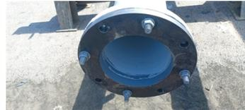
Flange face repair by flange face forming technique in progress
