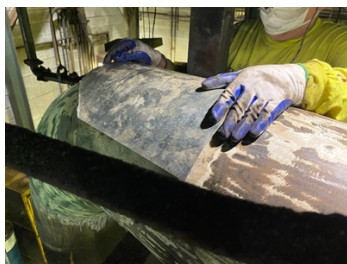
Cold Bonding Former with Belzona 1212
