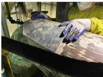
Cold Bonding Former with Belzona 1212
