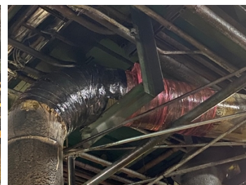
Finished Application (Consolidation Tape still needs removed)
