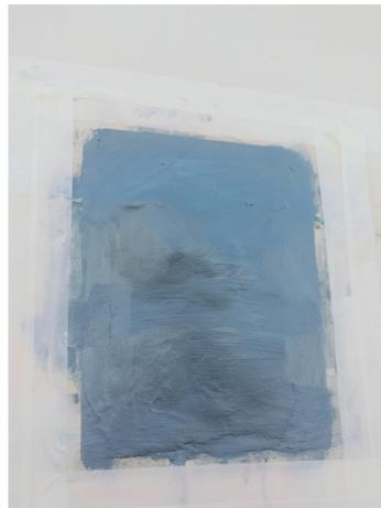
To strengthen the repair area, Belzona 1161 (Super UW-Metal) was applied before proceeding with plate bonding.
