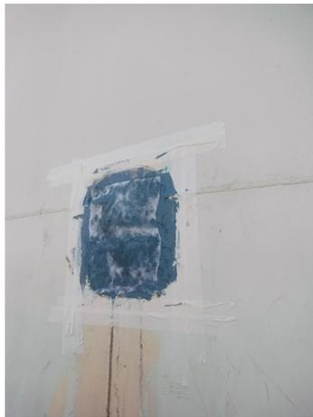
Following cleaning, the substrate was grit-blasted, and Belzona 9611 (ES-Metal) was applied to effectively seal the leak.
