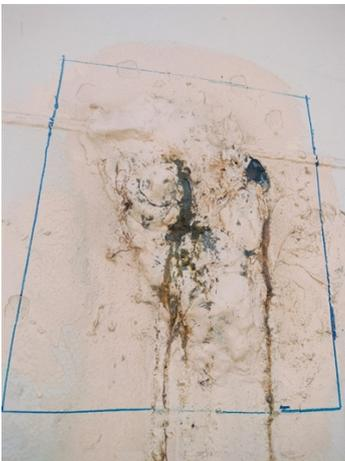
A leak in the wall of the customer's fire water tank created a hole and disrupted operations.
