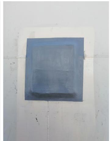
Belzona 1161 (Super UW-Metal) was applied via the plate bonding method.
