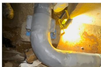
In this photo we show how ,after we put the plates and the jubilees with the Belzona 1212, we sealed all off with Belzona 1212 and Belzona 1161.
