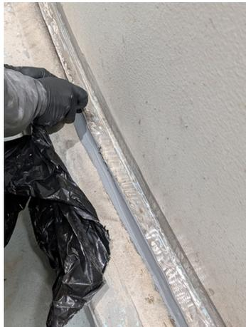
Stemming the leak with Belzona 1161
