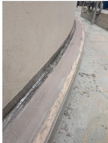
Sealing the perimeter with Belzona 4111
