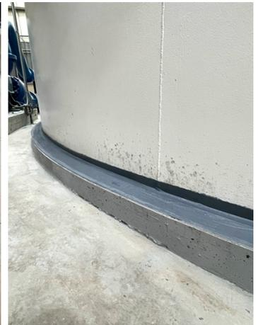
After application of two coats of Belzona 3111 with mesh.
