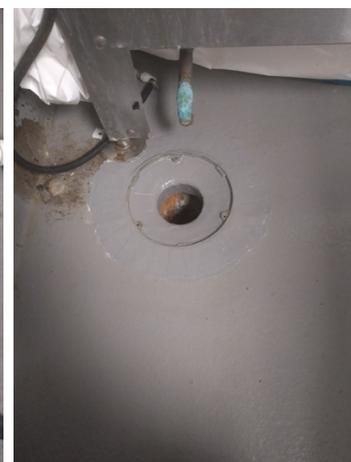
Ice machine with drain below
