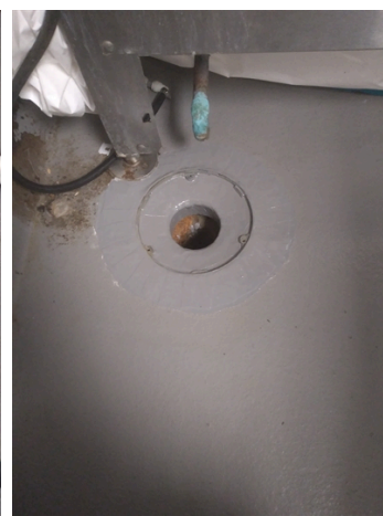
After application was completed with Belzona 3121
