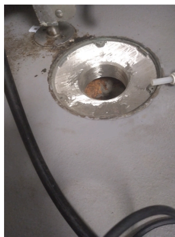
After surface prep was completed SSPC-SP11
