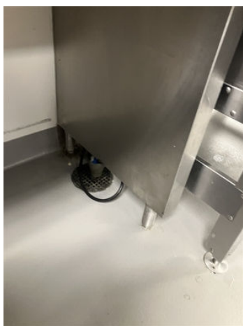
Ice machine with drain below
