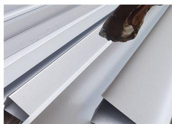
New pre-fabricated gutter linings ready to be bonded over the existing failed substrate with Belzona 1161 then coated with Belzona 3111.
