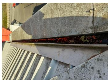
Gutter above concourse, showing corrosion, failed joints and dropped edges.
