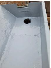
Completed downpipe end, ensuring that all joints, welds and seams were perfectly encapsulated.
