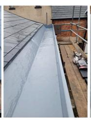
Particular attention was paid to Application of Belzona 3131 system completed, returning the gutter to watertight and alleviating the issues to the shop owners.
