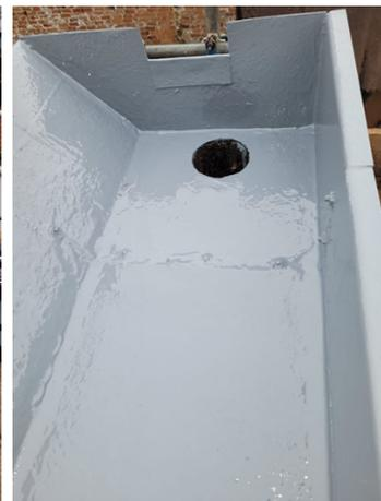
Gutter cleaned and prepared using High Pressure jetting equipment.
