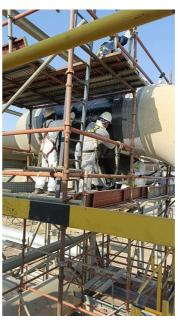
Application of the Belzona SuperWrap II system in progress.
