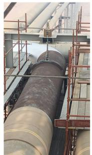
A 58" flare line in a petrochemical plant had suffered significant wall-thickness loss, compromising its structural integrity.
