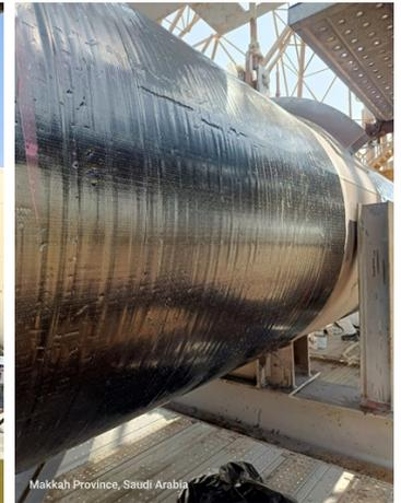
A 58" flare line in a petrochemical plant had suffered significant wall-thickness loss, compromising its structural integrity.
