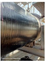
Completed application of Belzona SuperWrap II on the flare line.
