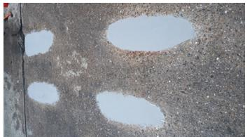
Showing landing legs causing wear to concrete parking area near loading doors
