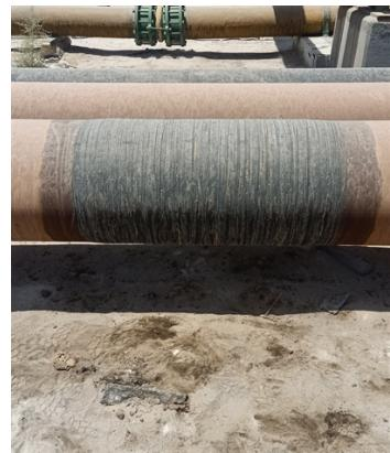
The 20" pipe was clamped by the customer due to severe leakage.
