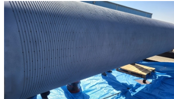
Surface preparation prior to the application of Belzona 1391T
