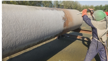
Surface preparation prior to the application of Belzona 1391T
