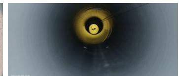
Condition of the substrate after grit blasting and before internal coating application.
