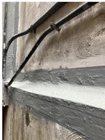
This is a close up on the 3121/9331 repair on the horizontal and vertical joints, after the job was completed.
