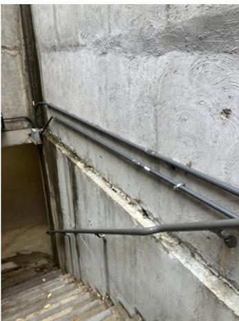
This image shows the leak externally in the vertical and horizontal joint of the wall.
