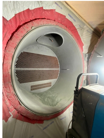
After the abrasive blasting was completed, SSPC-SP10.
