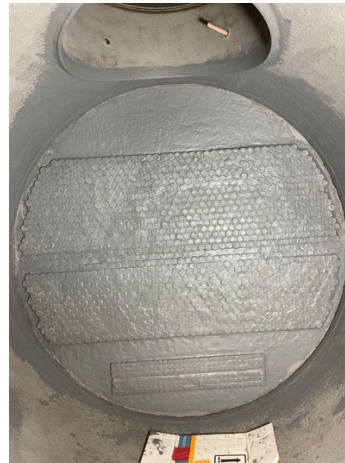
After Belzona 1121 was used to pit fill the tube sheet.
