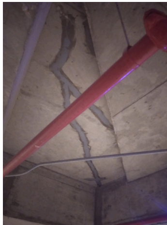
Belzona 9611 and 1212 used to composite patch crack and stop the active leak.
