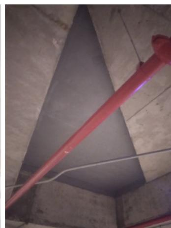
Entire ceiling area sealed with Belzona 3121 and 9331
