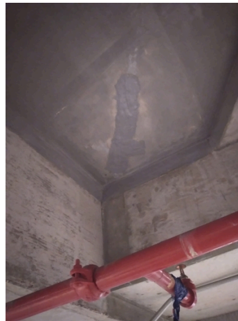
Belzona 3121 and 9331 applied to patch the crack and perimeter seams.
