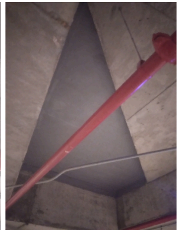
Entire ceiling area sealed with Belzona 3121 and 9331
