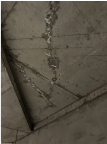
Long crack in the ceiling of the garage, before image.
