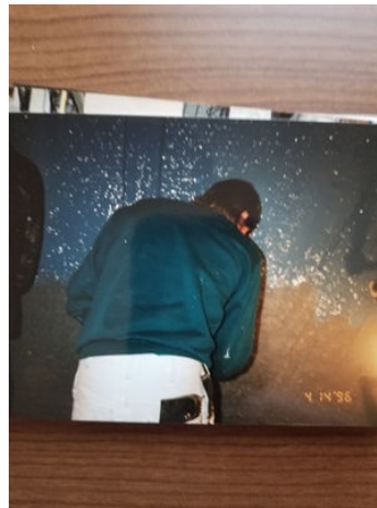
Application of 2 coats of Belzona 1321
