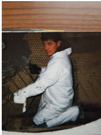
Contractor applying Belzona 1121 between all tubes; bring it flush with tubes
