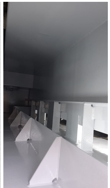
Completed application of Belzona 5892 system
