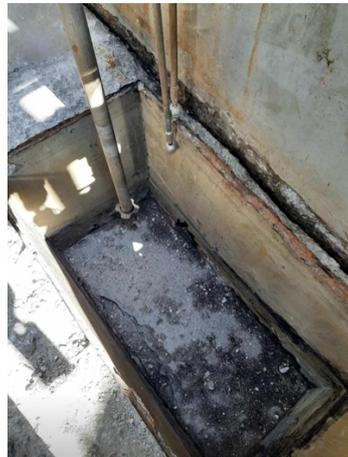
Close up of the sump pit area. Here you can see how bad the concrete had deteriorated between the sump pit and exterior wall of the containment.
