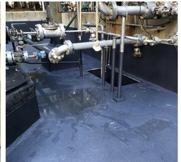
Once the repair was complete we applied 2 coat of Belzona 4311. In this application we perform a yearly inspection for the client.
