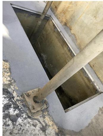
In this picture, after we removed all loose and damaged concrete we thoroughly cleaned the area to be repaired with 100% MEK and began to prep the surface with grinders and needle guns. Once we achieved the correct surface prep we applied Belzona 4111
