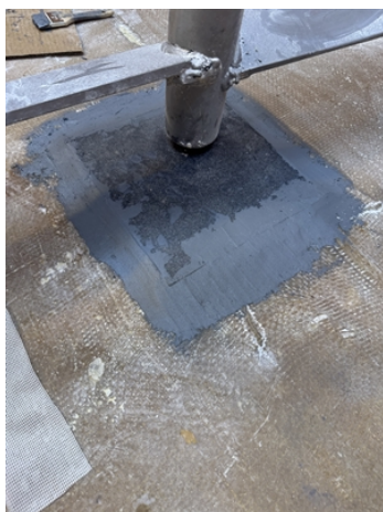
Belzona 1111 with Reinforcement Cloth shown over a cold plate bond on floor of fiberglass tank
