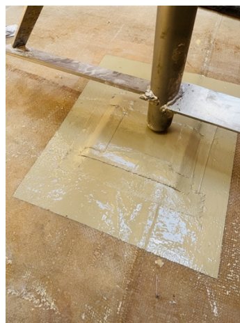
Belzona 5815 and Composite Reinforcement Wrap Overlay on 1111 Repaired Areas
