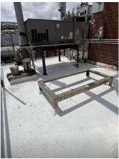
You can see in this photo the water standing due to poor slope and deep pitting in the concrete caused from deterioration.
