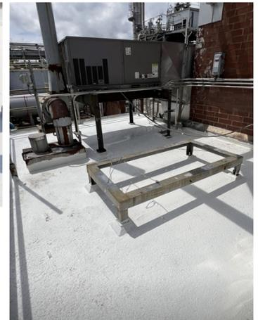
You can see in this photo the water standing due to poor slope and deep pitting in the concrete caused from deterioration.
