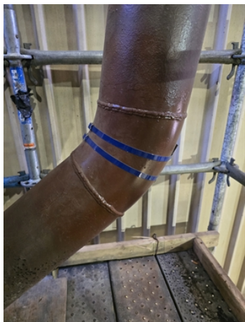
Fly ash elbow with temporary patch.
