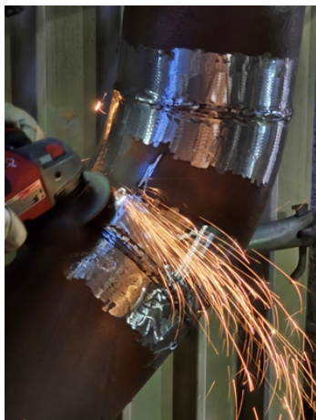
Removing the paint and prepping the surface.
