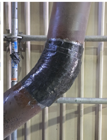
Belzona SuperWrap II applied over the Belzona 1813 and the elbow.
