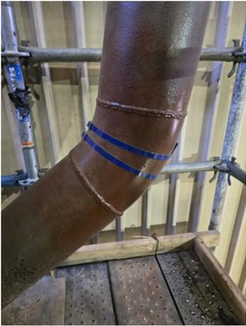
Fly ash elbow with temporary patch.
