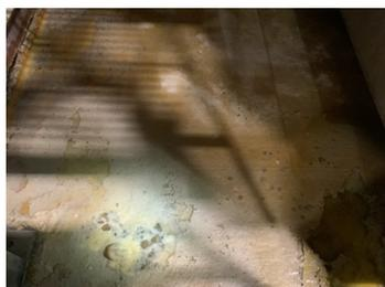
A close up view of the old coating and how it is delaminating.
