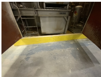
This photo shows you how we cleaned and removed the old coating and prepped the surface area to be coated.
