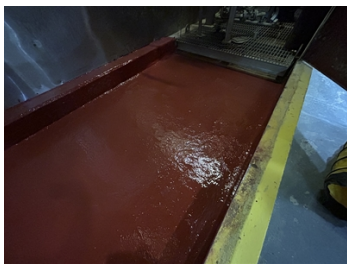
Final photo shows the completed project using Belzona 4111 and Belzona 4311.
