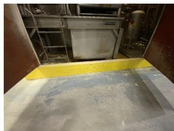
This photo shows you how we cleaned and removed the old coating and prepped the surface area to be coated.
