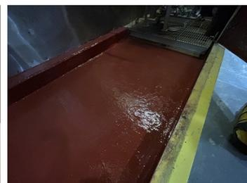
Final photo shows the completed project using Belzona 4111 and Belzona 4311.
