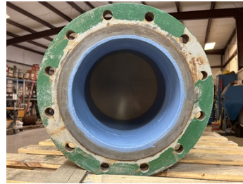
After blasting to a 3 mil profile and first coat of Belzona 1321
