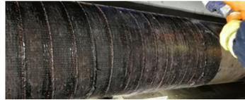
Up close of applying Belzona 1984 and Super Wrap II
