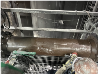
Removing build up and rust before applying Belzona 1984.
