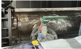
Prepping the surface with grinders and MBX Bristle Blaster.
