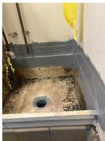
Mop sink showing water infiltration points around the drain and wall interfaces prior to repair. Gaps between the sink, walls, and drain allowed water to escape the basin and leak to lower floors.
