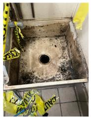
Mop sink showing water infiltration points around the drain and wall interfaces prior to repair. Gaps between the sink, walls, and drain allowed water to escape the basin and leak to lower floors.
