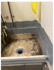
Completed repair using Belzona 3121 (MR7), creating a directing water into the drain and preventing further leakage.
