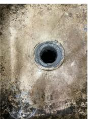
Close-up of the drain penetration sealed using Belzona 3121 (MR7) to prevent continuous waterproof seal water migration around the pipe connection.
