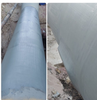
Pipeline condition following plate bonding using Belzona 1221 and wrapping with Belzona 1161 (Super UW-Metal) and Belzona 9341
