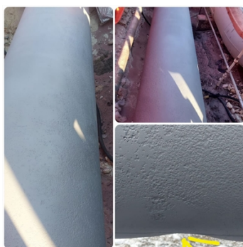
Pipeline condition after surface preparation by grit blasting
