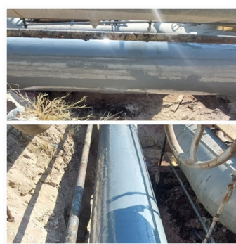
Pipeline condition following application of Belzona 5831 (ST-Barrier) for external corrosion protection
