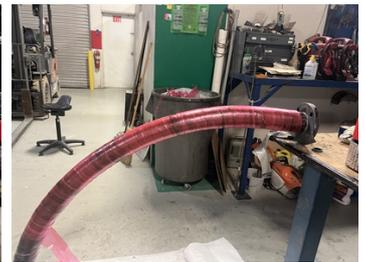
Completed wrap after applying the consolidation tape.
