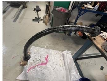
Applied Super Wrap II using Belzona 1984
