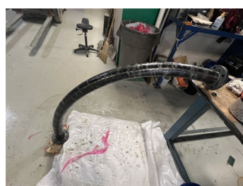
Applied Super Wrap II using Belzona 1984
