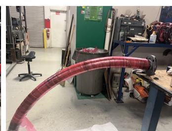
Completed wrap after applying the consolidation tape.
