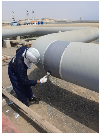
Application of Belzona 1111 (Super Metal) and Belzona 9341 (Reinforcement Tape) conventional wrapping in progress.
