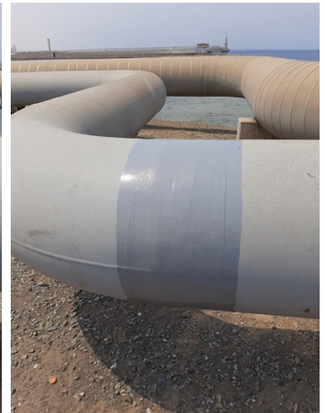
Completed application of the Belzona conventional wrapping system.
