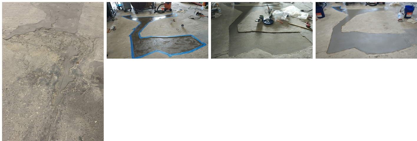
Damaged sections of the floor After surface preparation, the area was conditioned with Belzona 4911 The area was filled with Belzona 4124 except for the top 1/4 inch Top 1/4 inch was filled with Belzona 4131
