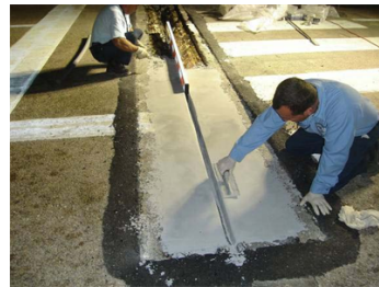
Expansion joint nosings being rebuilt with Belzona 4111
