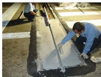
Expansion joint nosings being rebuilt with Belzona 4111
