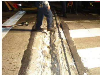
Surface preparation completed
