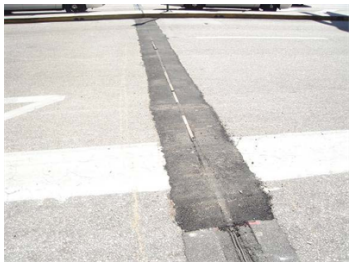
Existing expansion joints
