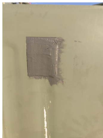
Application of Belzona 1212 with Belzona 9341 Reinforcement Tape
