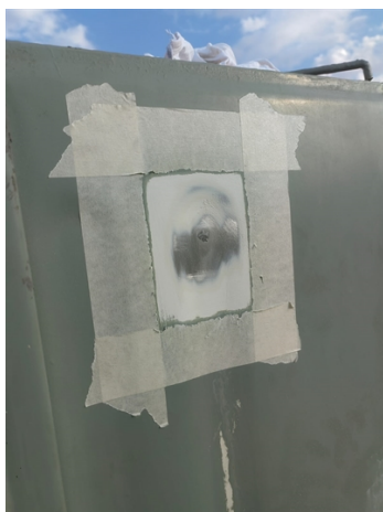
Surface Preparation of the Leakage Area
