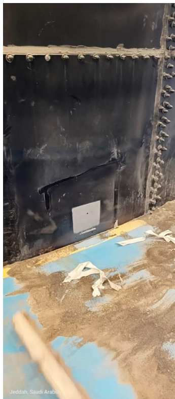
Surface preparation carried out by grit blasting
