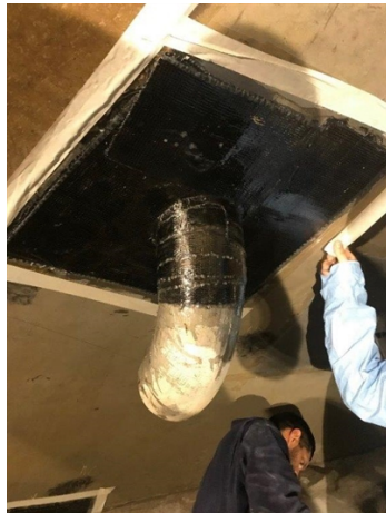
Area was blasted with aluminum oxide and Super Wrap II applied.
