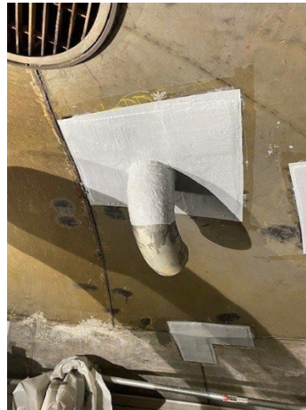
SuperWrap II was top coated with Belzona 5811 and 5111.
