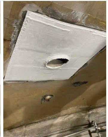
Secondary area completed with SuperWrap II and top coated with Belzona 5811 and 5111.
