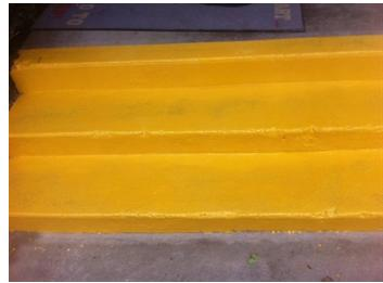
Worn Belzona 5231 areas from an application applied in January of 2000.
