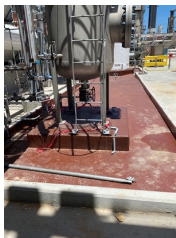
Completed secondary containment area.
