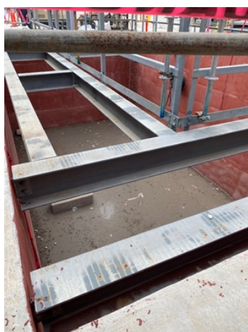
Dump pit halfway completed with Belzona 4181 AHR Magma Quartz.
