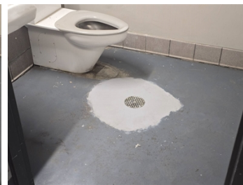
Application of Belzona 4111
