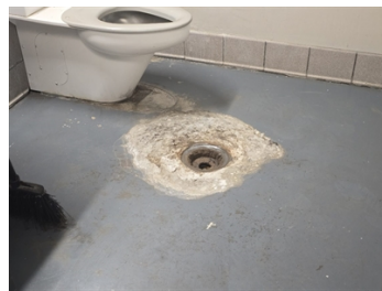
Removal of previous patch material
