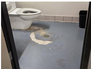
Condition prior to repair
