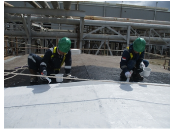
Application of Belzona 3111 (Flexible Membrane) in conjunction with Belzona 9311 (Reinforcement Sheet).
