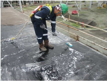
Surface cleaning was carried out to prevent contamination.
