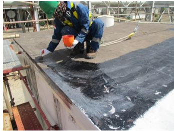
Belzona 3911 (PSC Surface Conditioner) was applied.
