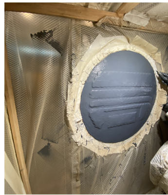
Application of Belzona 1311 and Belzona 1321.
