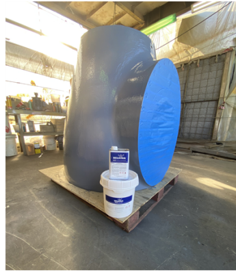
Belzona 5821 First Coat
