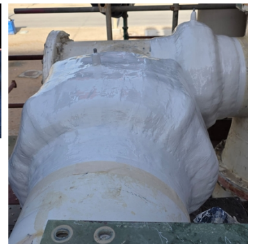
Application of Belzona 5721 UV-resistant topcoat.
