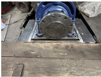
Bearing Foundation Set and Aligned
