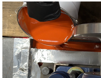
Belzona 7111 Being Poured Into Foundation
