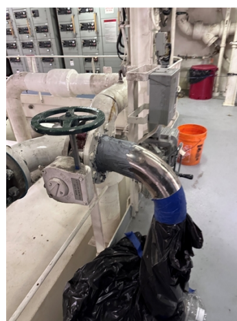
Belzona 1161 Being Applied
