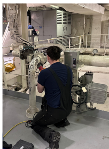
Temporary Repair Made at Sea Surface Prep
