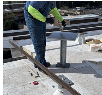
Applying Belzona 4911 Surface Conditioner
