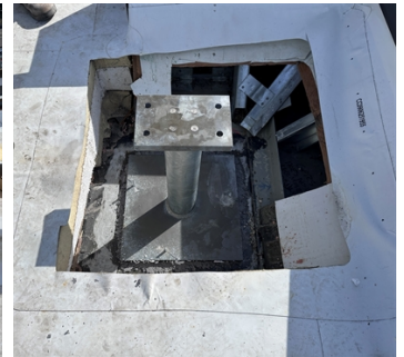
Final Application with 1/4" of Belzona 4111
