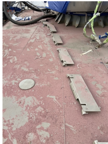
Surface preparation work underway on the vessel deck
