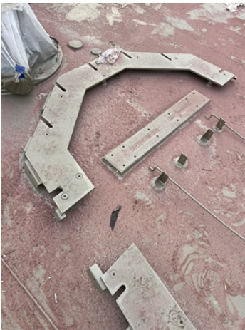
Surface preparation on the vessel deck in progress
